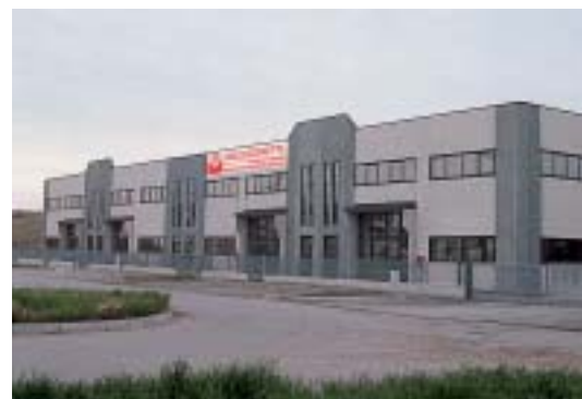
Secondo magazzino scorte/ Second stock warehouse
